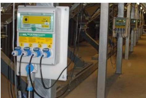
Static units control any quantity of ventilation fans. Portable units can be moved with fans and are simple to install.
