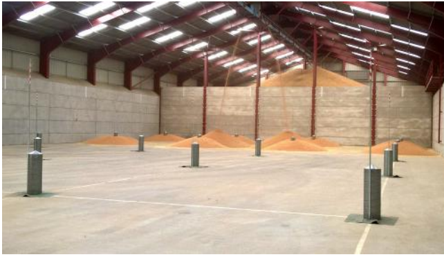
FloorVent Pedestals - ideal for large, deep grain stores
