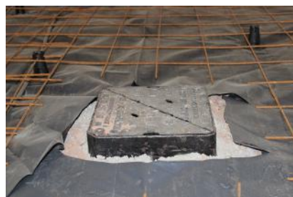
Installation uses standard building materials
