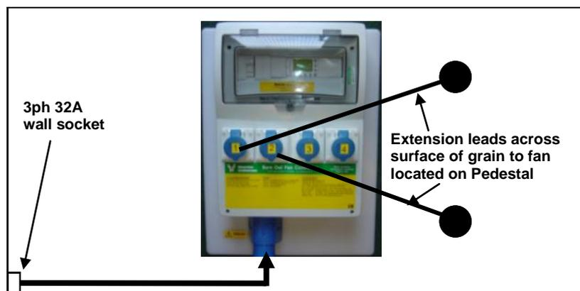
Recommended electrical and socket requirements for connection of a board-mounted controller to Pile-Dry Pedestal Fans is as follows:
